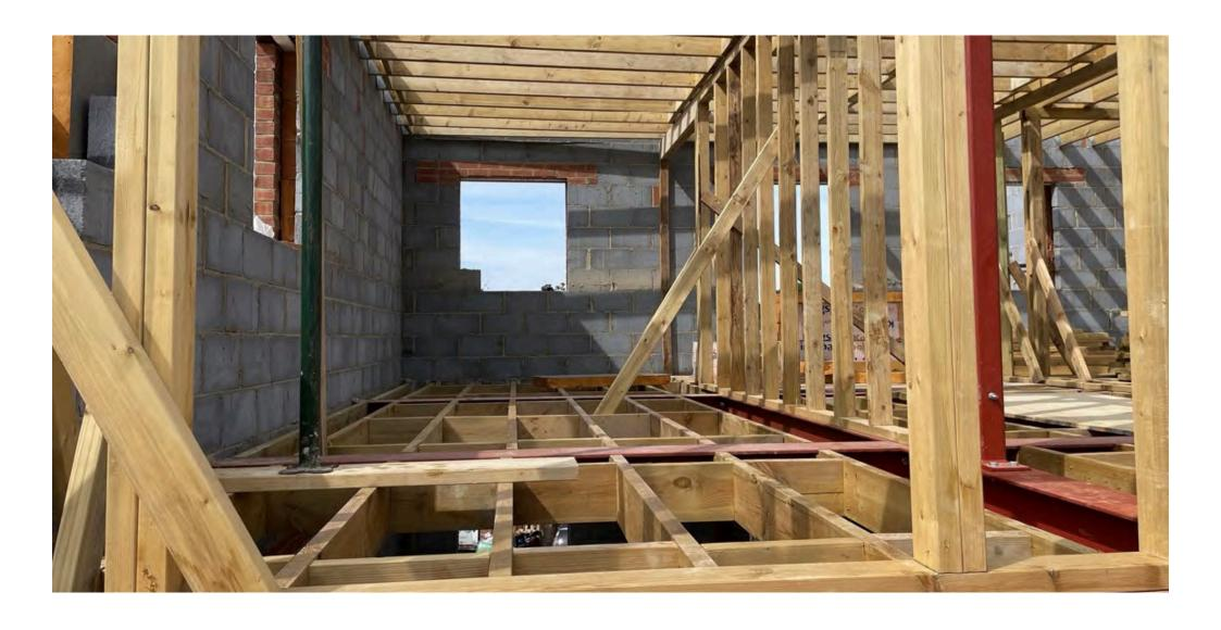
On the other two floors the stud walls are being put in place ready for plasterboard and plastering.
