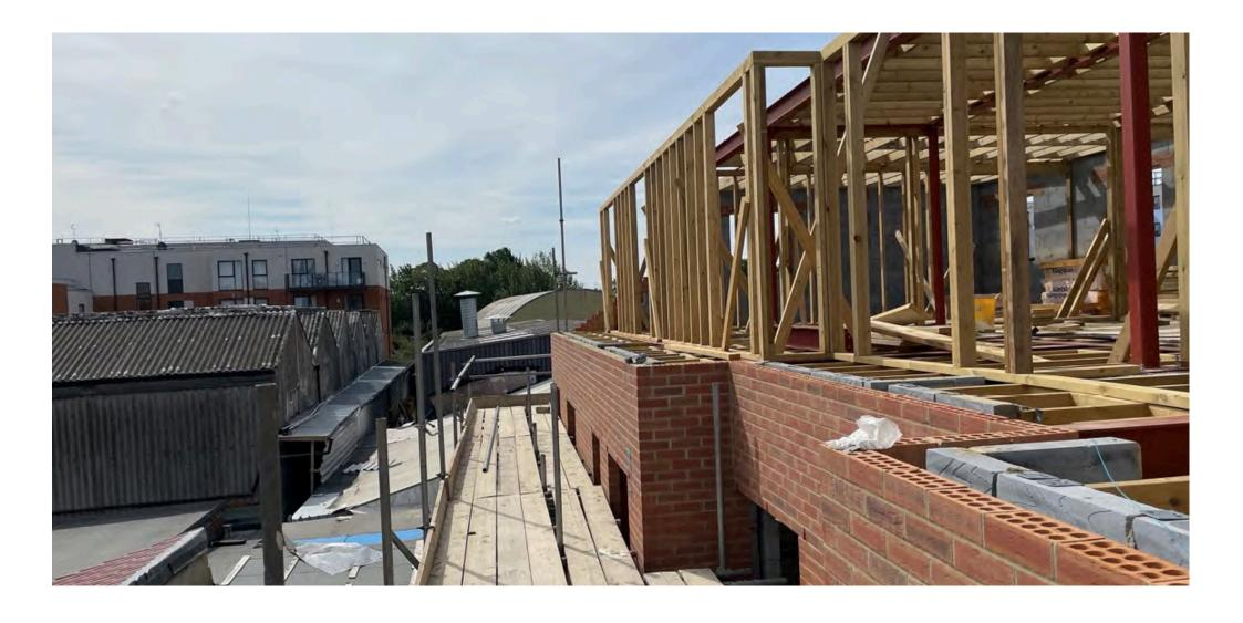
The last few layers of bricks have been added to the rear of the building which will enable the flat roof to be completed.
