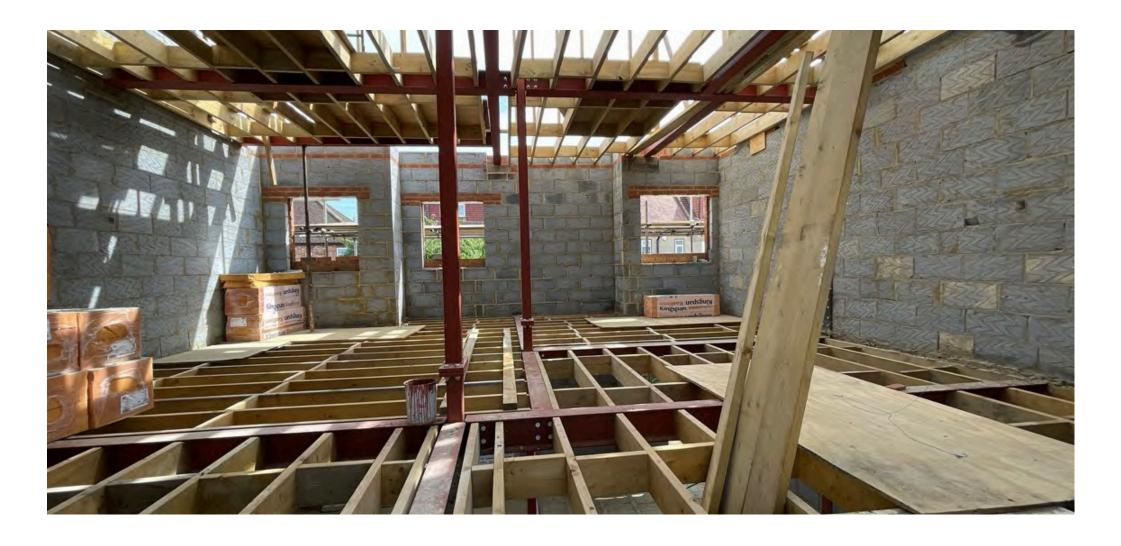
On the First Floor the first fix is being done and the insulation will be installed soon.
