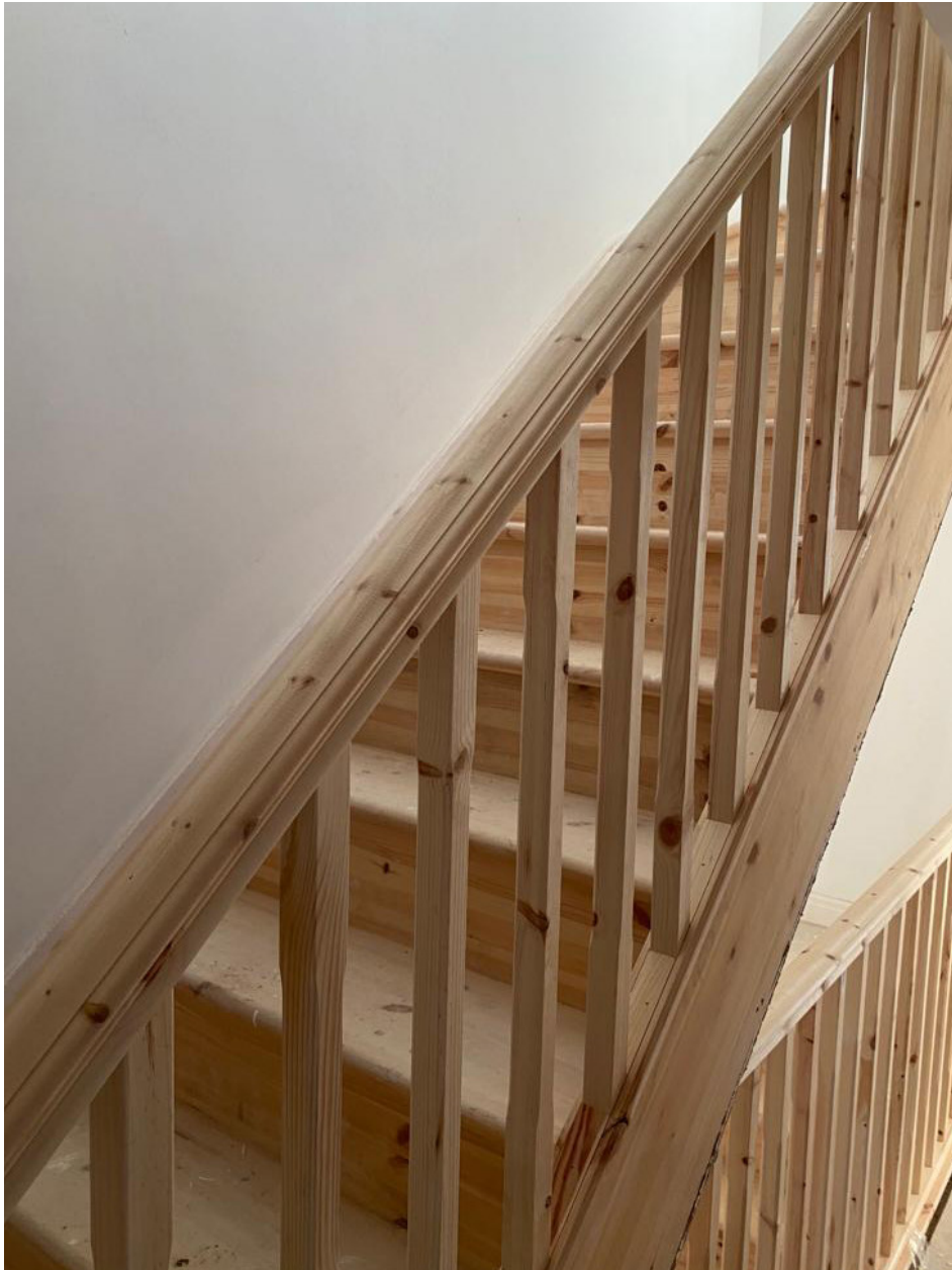
Some of the staircases and balustrades are in place.
