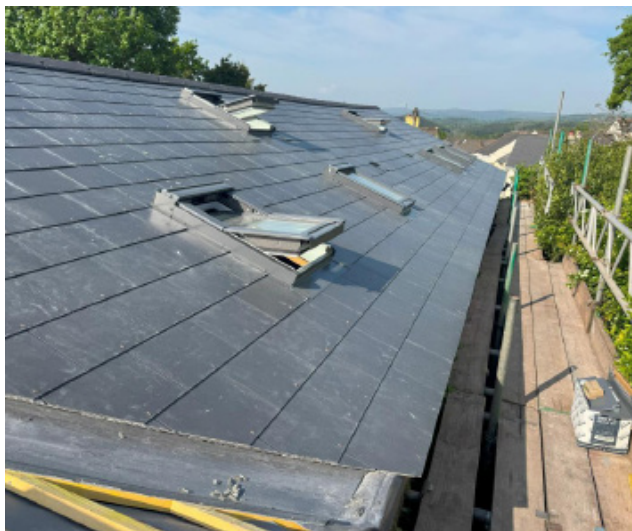
Roofing works and velux windows installations
